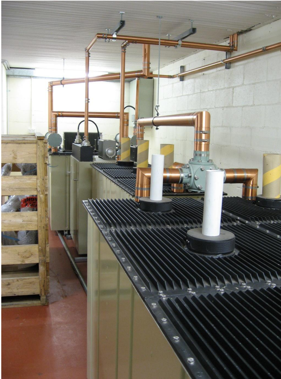
192. Downstairs at Broadcasting Park, Mount Coot-tha. The combiner system that joins the five station's signals into the one antenna. Photo: © Gavin Unsworth 2007.
