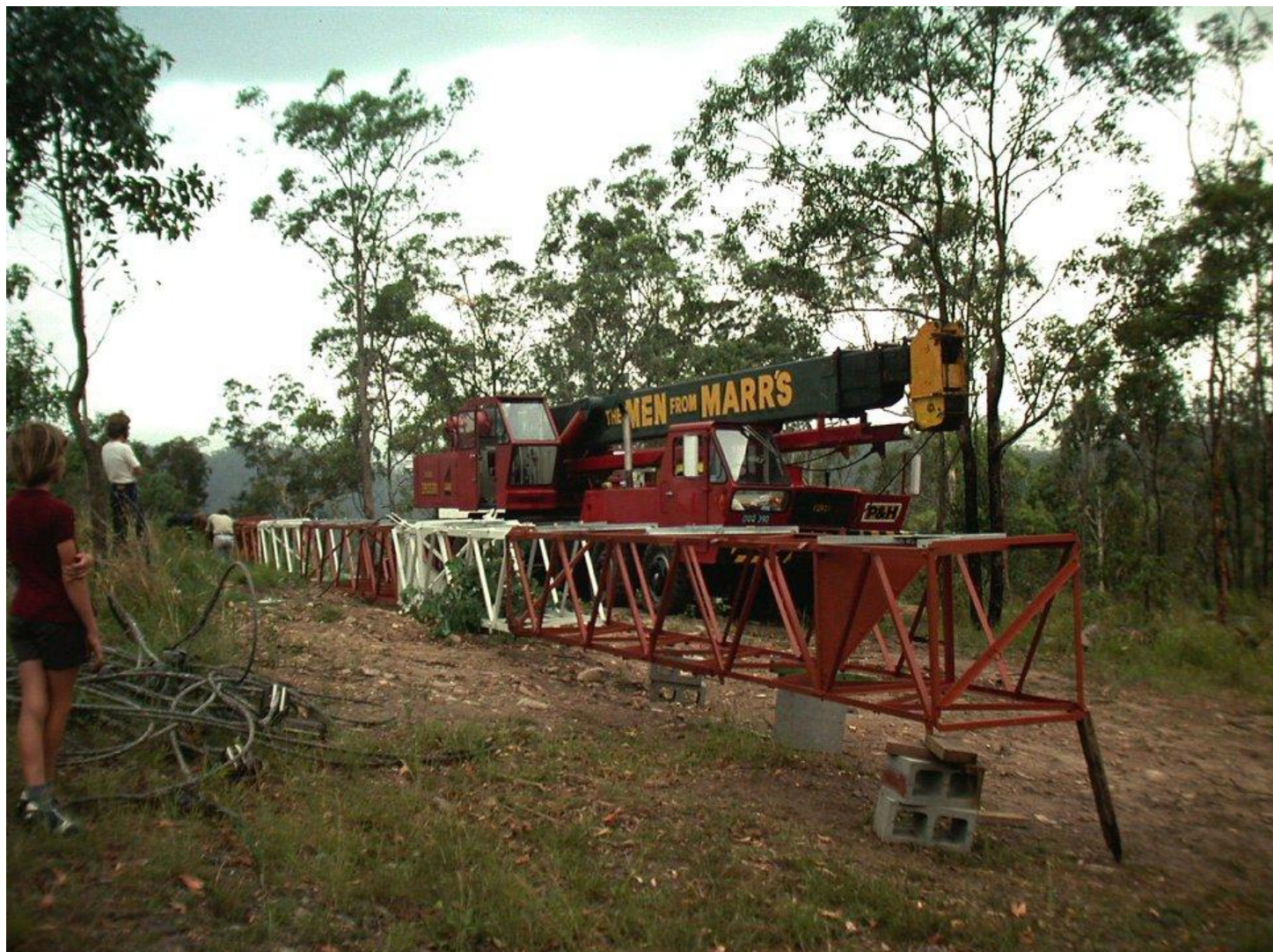
78. This tower was relocated from an AM radio transmitter site that had to be removed because of extensions to the Brisbane airport. It was taller than needed, so they removed 30 feet from the top which left a 90-foot mast on which to mount the 4ZZZ antenna. Photo courtesy of Gavin Unsworth (4ZZZ radio engineer). (20 October 1977, photographer unknown)
